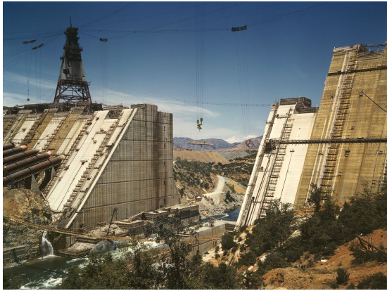
[Construction of Shasta Dam]
