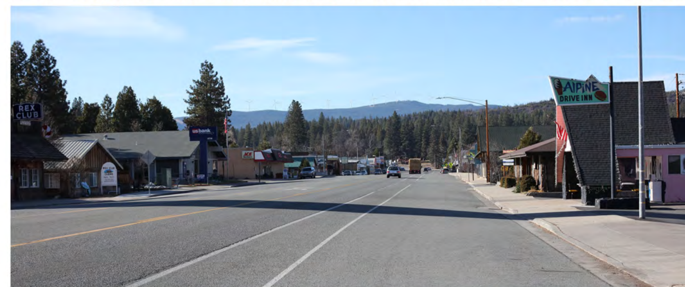
5. View to southwest from downtown Burney. Nearest turbine location is 7 mi away.
