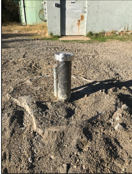
Photo 12 – Completed Test Well
