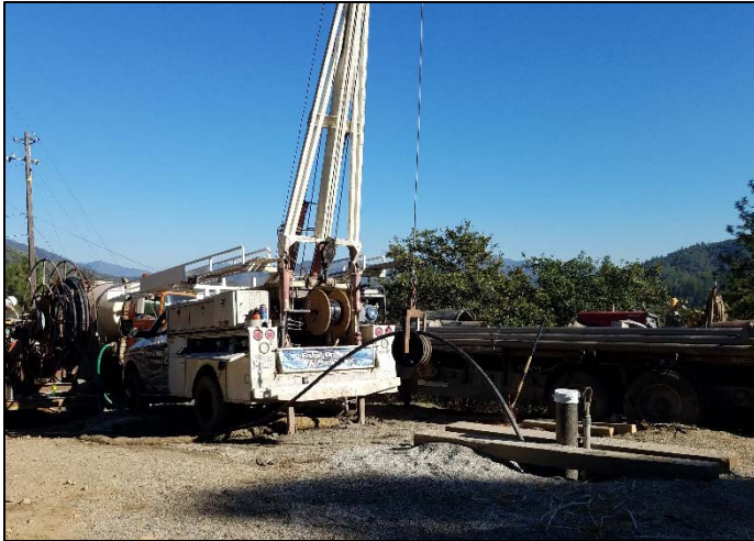
Photo 11 – Test Well Drilling
