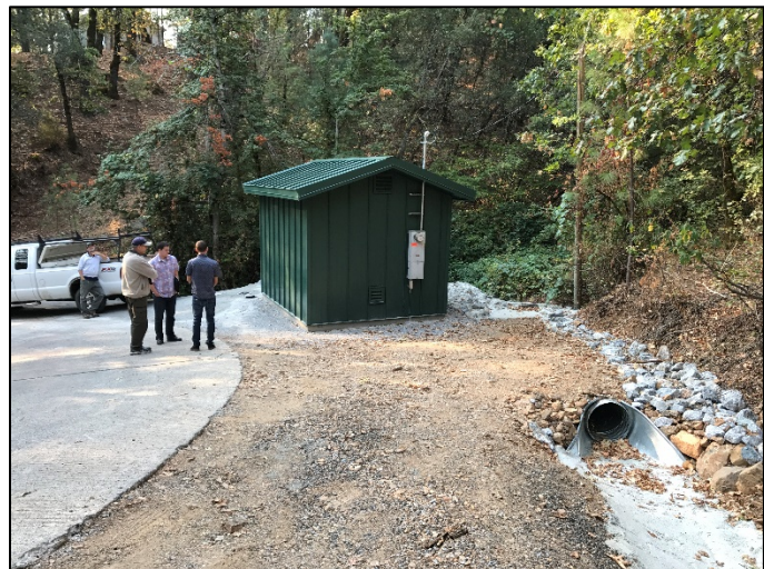
Photo 3 – Improved Existing Shale Lane Well
