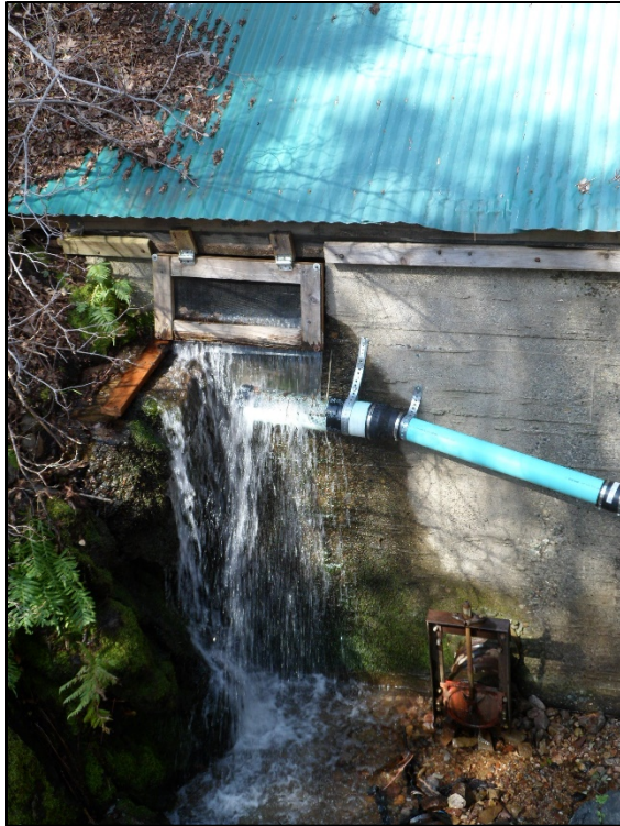
Photo 4 – Spring Diversion Dam
