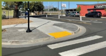
Curb Ramps/Curb Extensions
